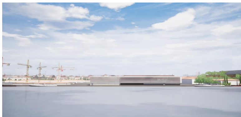
Figure 3.1. Panoramic view of the foundry
