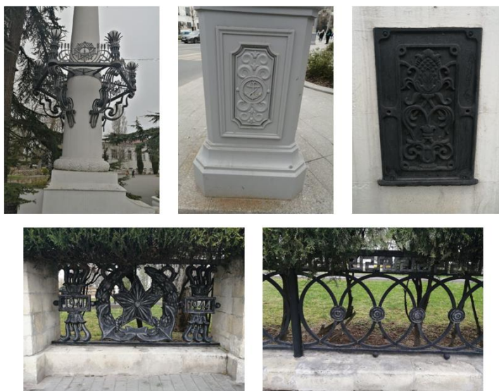
Figure 3.5. Photo fixation of the fragments of the Nakhimov Avenue design code
