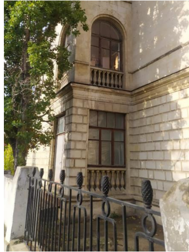
Figure 1. The facade of the Polytechnic Institute Building
