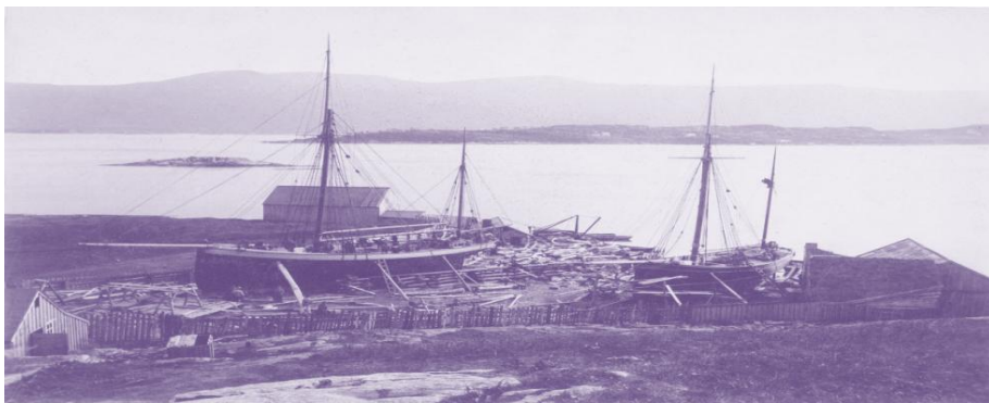
The building of Trio at the first shipyard on Ysteneset
